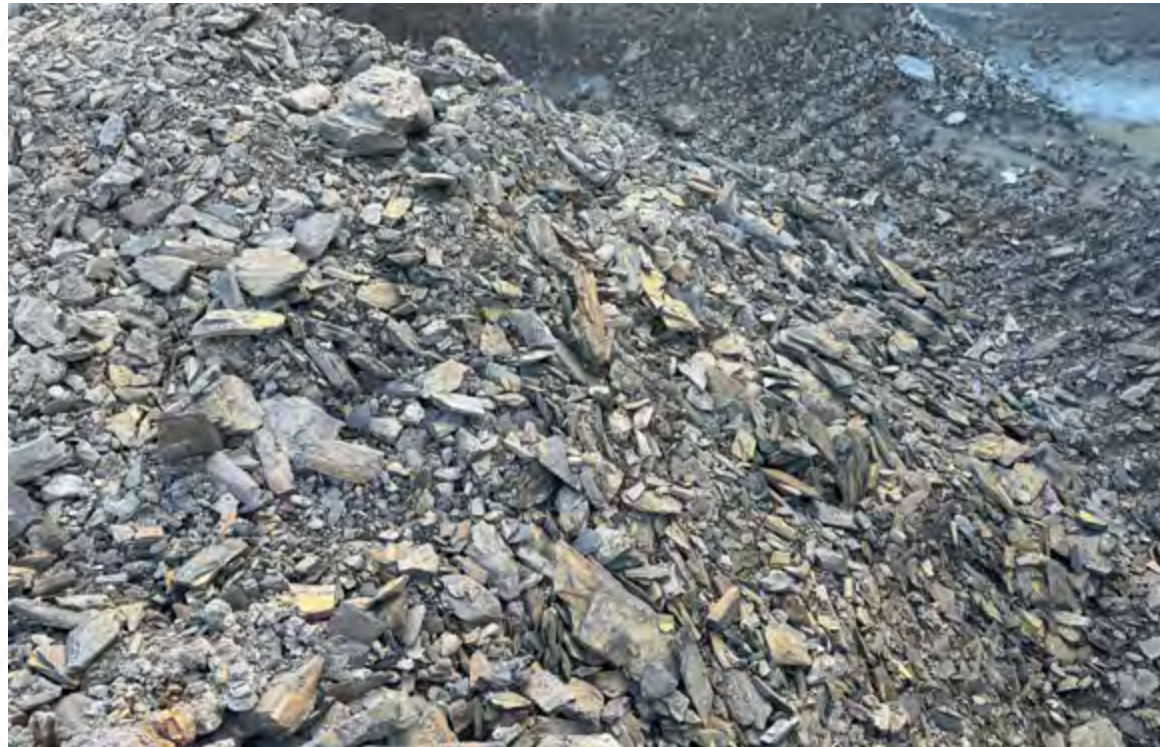
Shale Rock Foundation for stability
