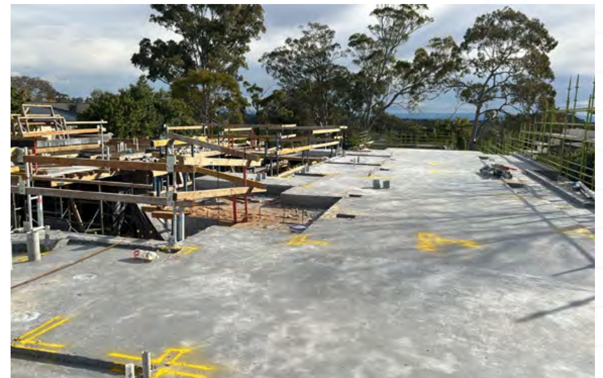
First Floor Concrete Slab
